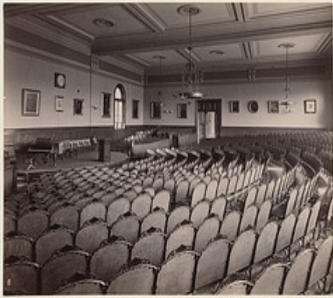
The General Assembly Hall has been prepared
